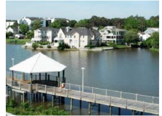
Lake Holly Pedestrian Bridge
