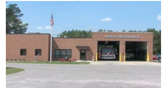
Driver Fire Station Addition
