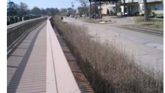
Haven Creek Bulkhead
