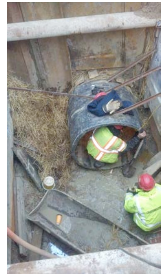
Pump Station No. 46 Force Main Horizontal Drilling
