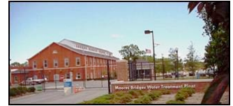
Moores Bridges Water Treatment Plant
