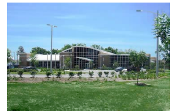
Lamberts Point Community Center
