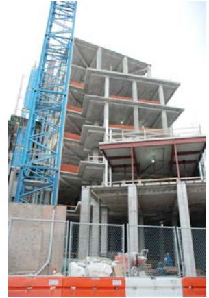
Slover Memorial Library Addition
