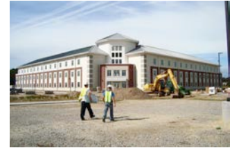
Thrun Hall Barracks, USCG Support Center, Elizabeth City
