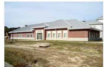
Thrun Hall Galley USCG Support Center, Elizabeth City
