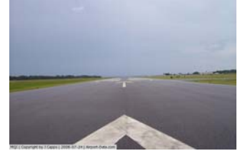
Taxiway, Dare County Regional Airport
