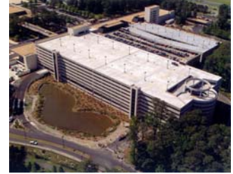
Parking Garage, Norfolk International Airport
