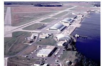
Hangar 6, USCG Support Center
